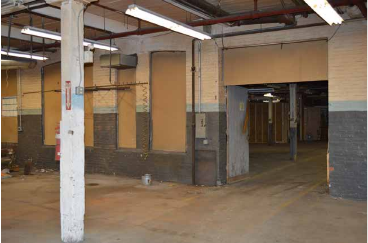
Building 2 addition interior
