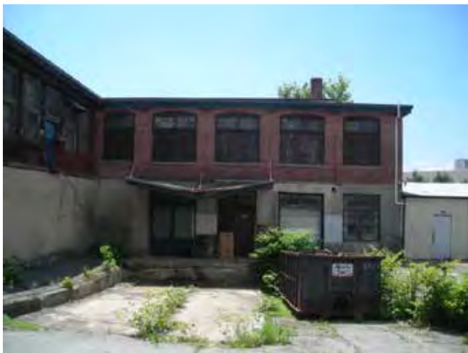
View south of loading dock at rear of Building 2 (left) and Building 1 ell (center)
