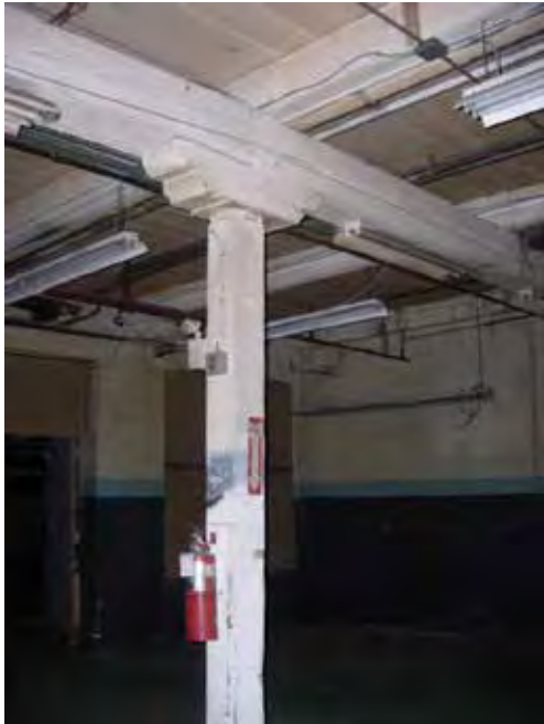
Building 2 addition, framing detail
