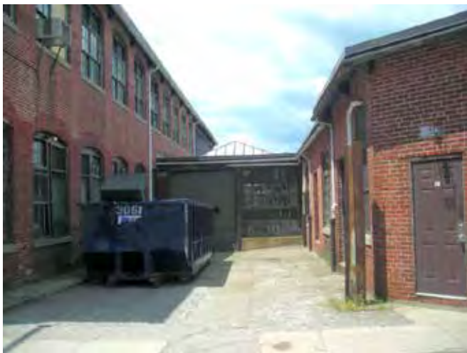
View west of loading dock between Building 1 (left) and Building 2 (right).
