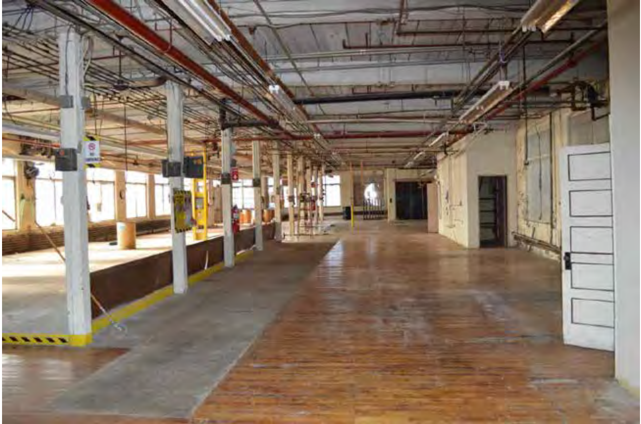
Building 1, Second floor
