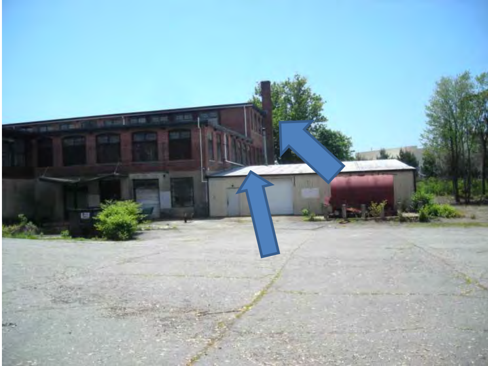
View south of rear of Building 1 and Building 4
