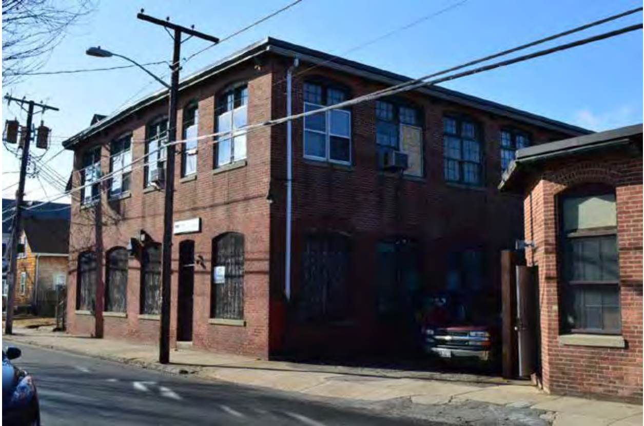
Façade of Building 1, view southwest
