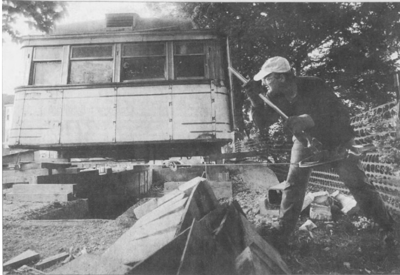
THOMAS COREY / THE HARTFORD COURANT COLIN STRAYER of Syracuse cranks a hand winch this week while working to move the former Farm Hill Diner, commonly known as "Squeaks." The 48-foot "Streamline" was built in 1941 by the Worcester Lunch Car Co. in Massachusetts and is one of only nine of its kind left in the country.
