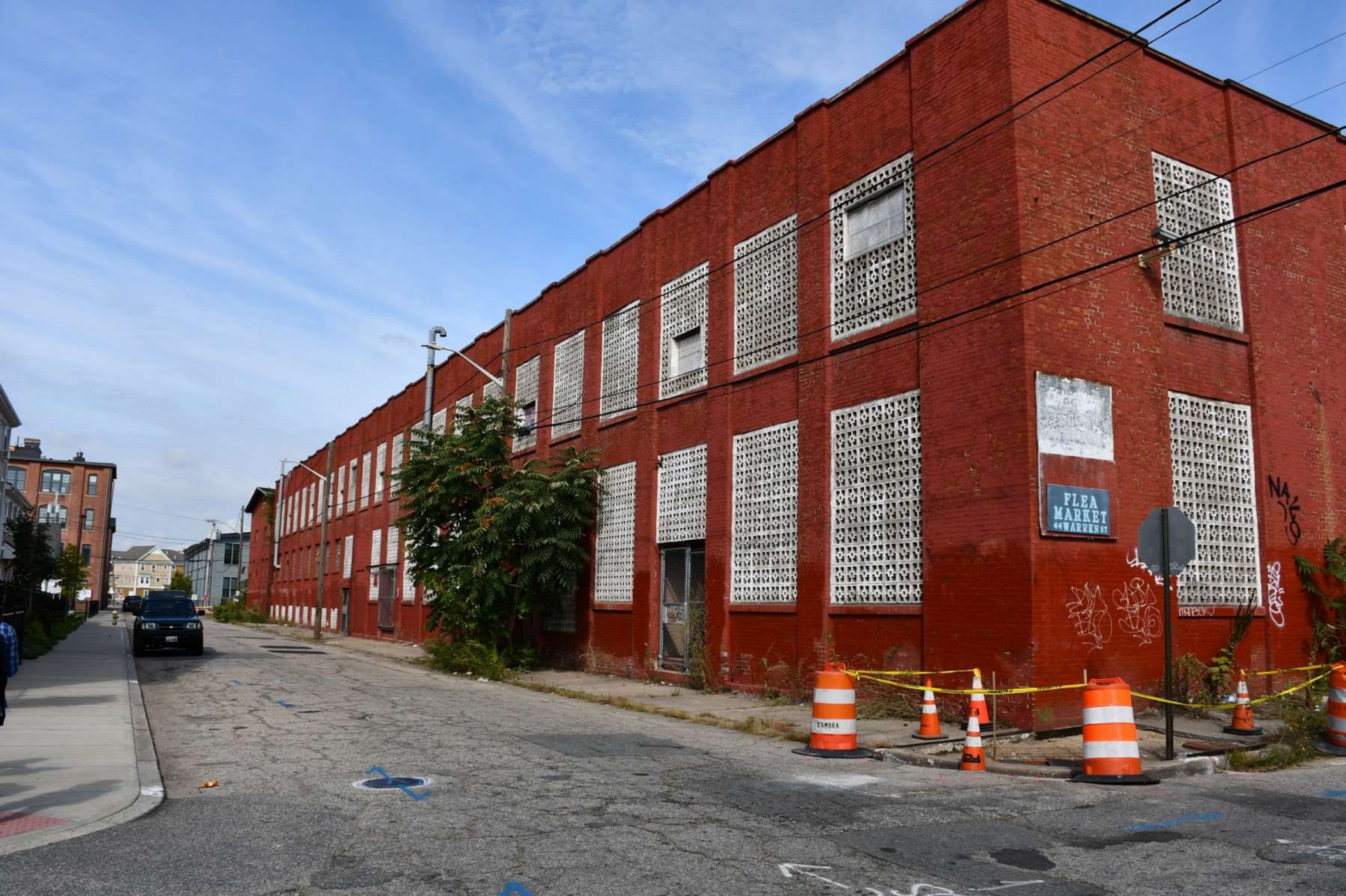
Photo #22 Building 3: Phillips Baker Rubber Company Building, south elevation facing northwest.
