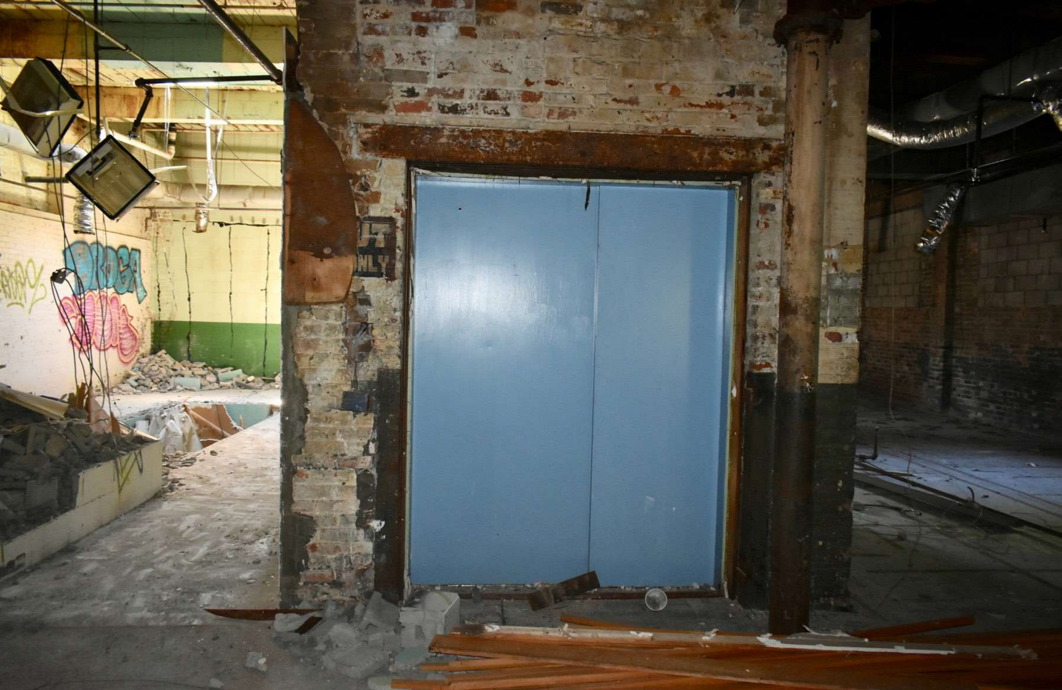
Photo #11 Building 1: Stedman & Fuller Manufacturing Company Building, second floor facing west.
