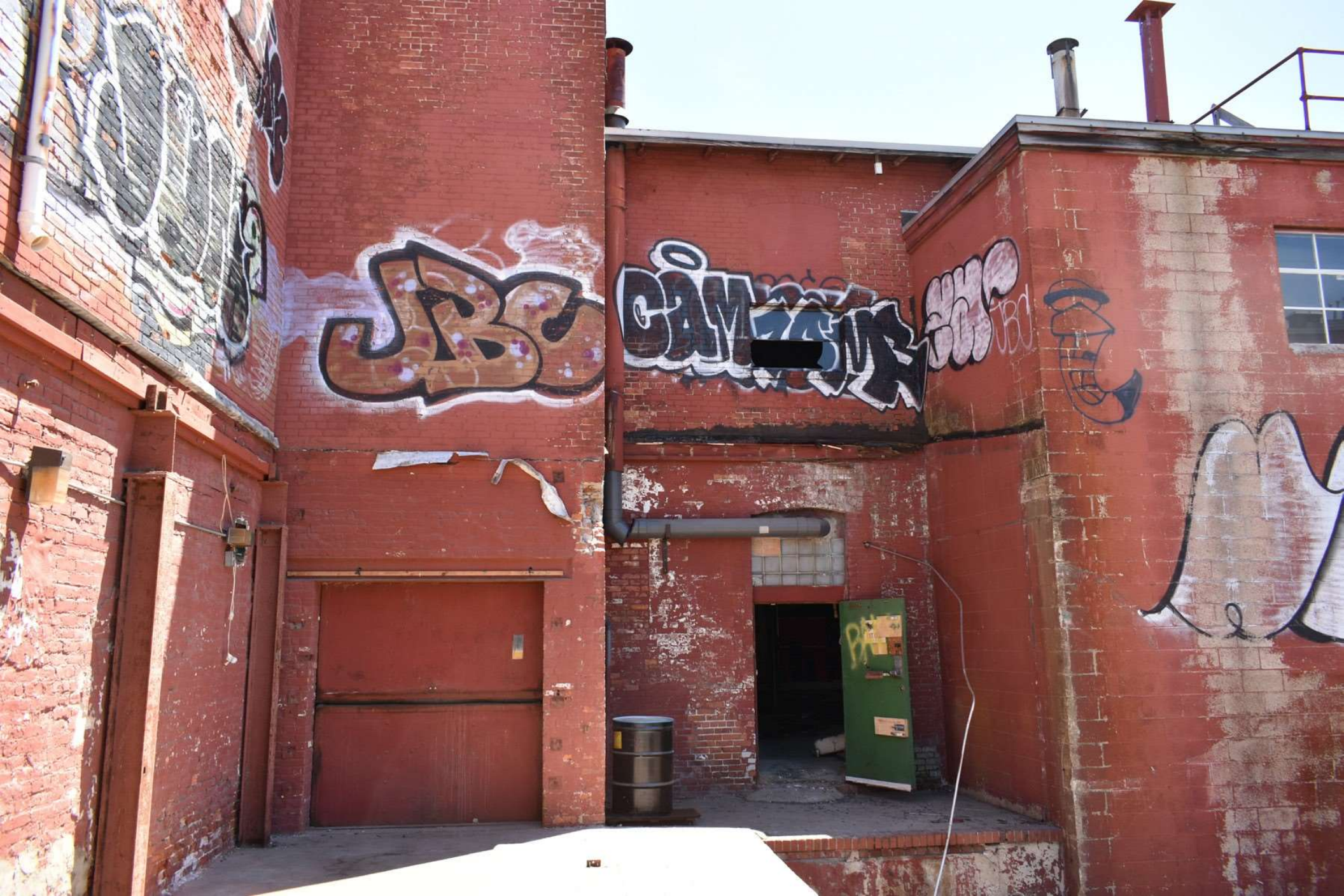
Photo #3 Building 1: Stedman & Fuller Manufacturing Company Building, west elevation, facing east.
