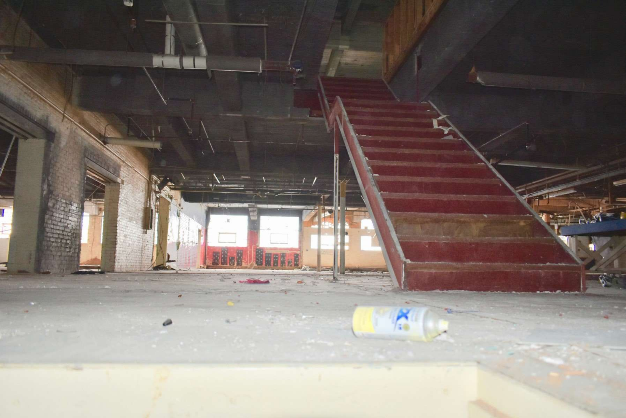
Photo #29 Building 3: Phillips Baker Rubber Company Building, first floor facing south.
