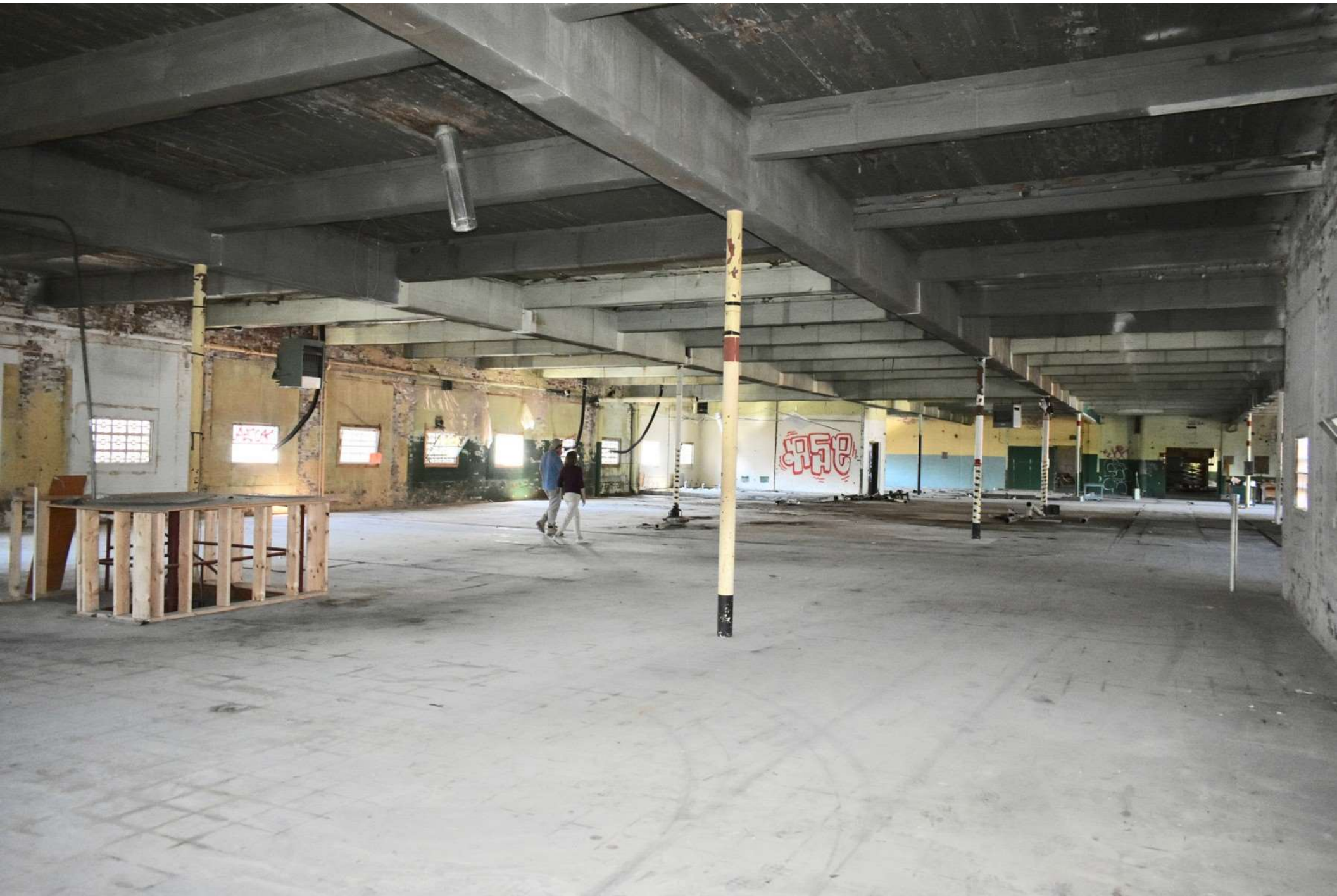
Photo #39 Building 3: Phillips Baker Rubber Company Building, second floor facing southwest.
