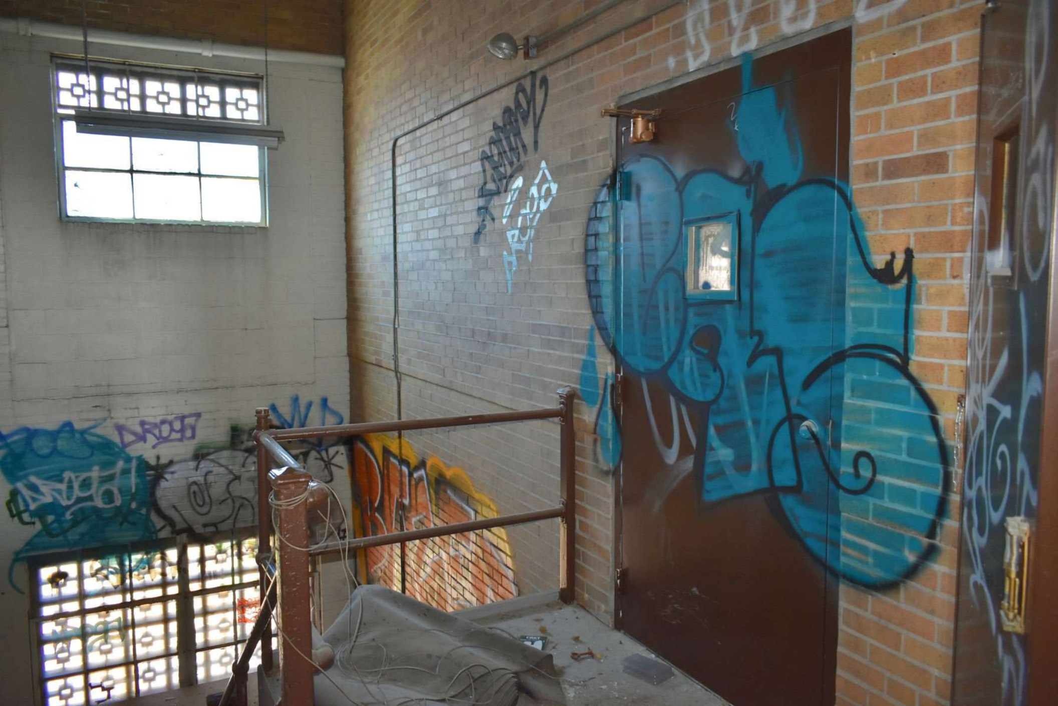
Photo #38 Building 3: Phillips Baker Rubber Company Building, second floor facing southeast.
