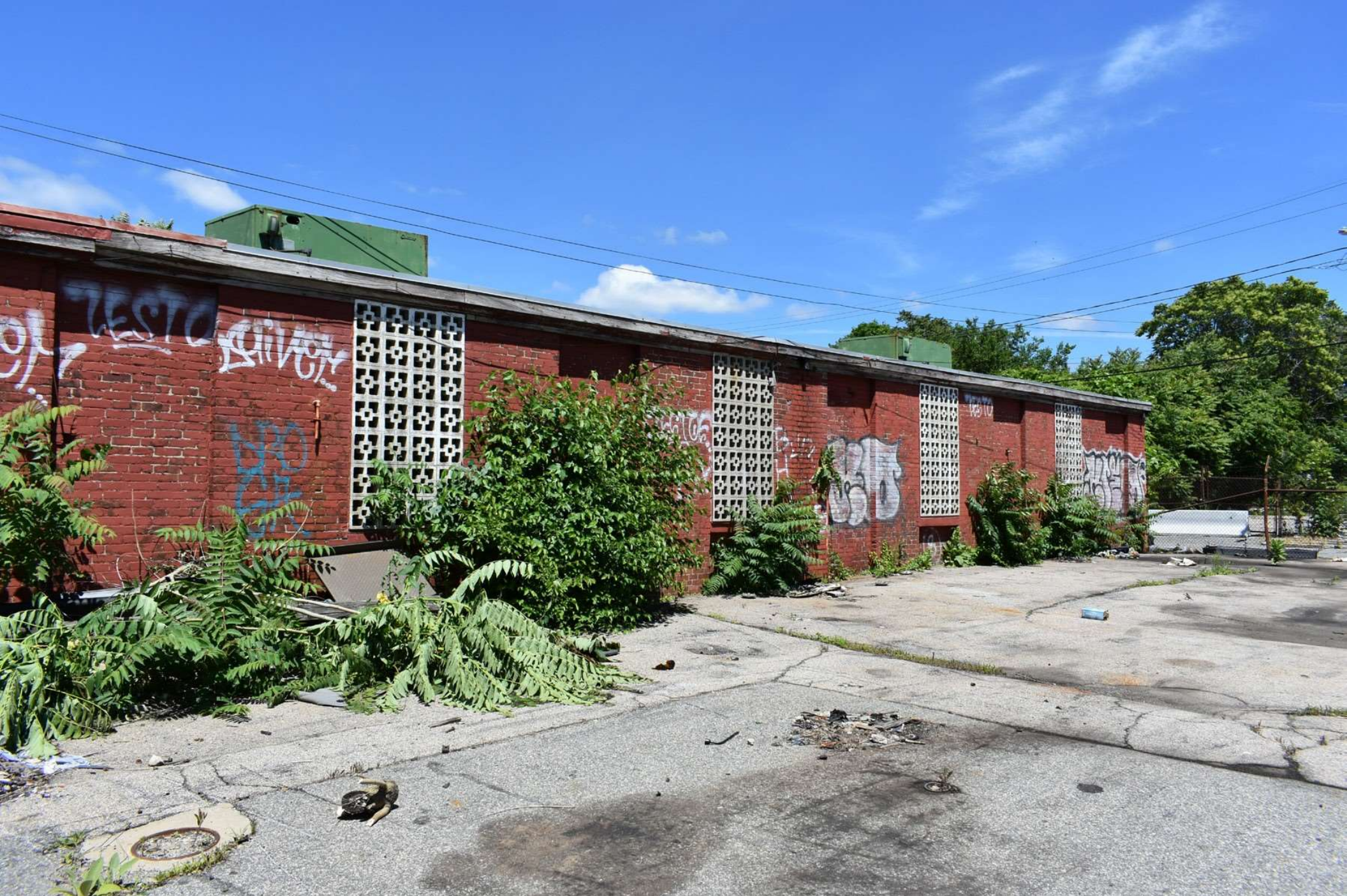
Photo #15 Building 2: Bourn Rubber Company Receiving Building, east elevation facing northwest.
