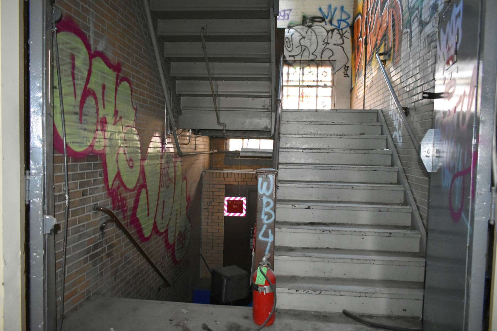
Photo #37 Building 3: Phillips Baker Rubber Company Building, first floor facing south.
