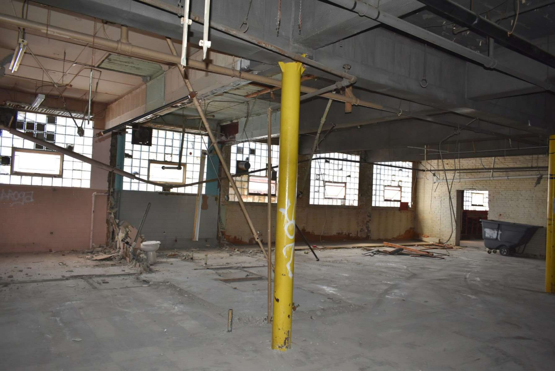
Photo #31 Building 3: Phillips Baker Rubber Company Building, first floor facing southwest.
