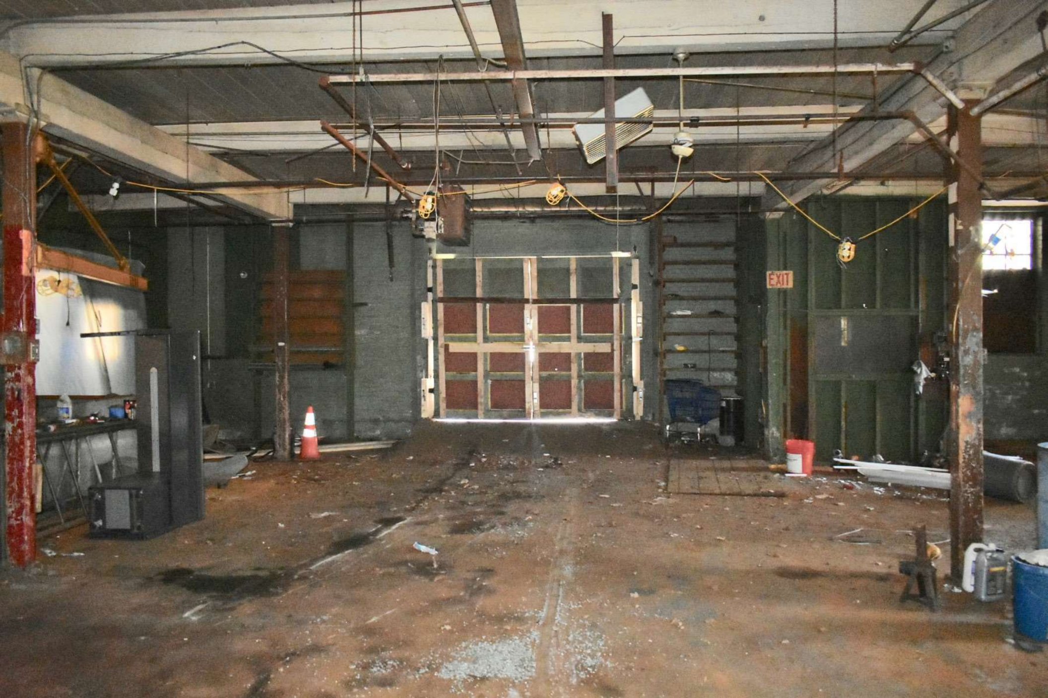
Photo #19 Building 2: Bourn Rubber Company Receiving Building, first floor facing north.
