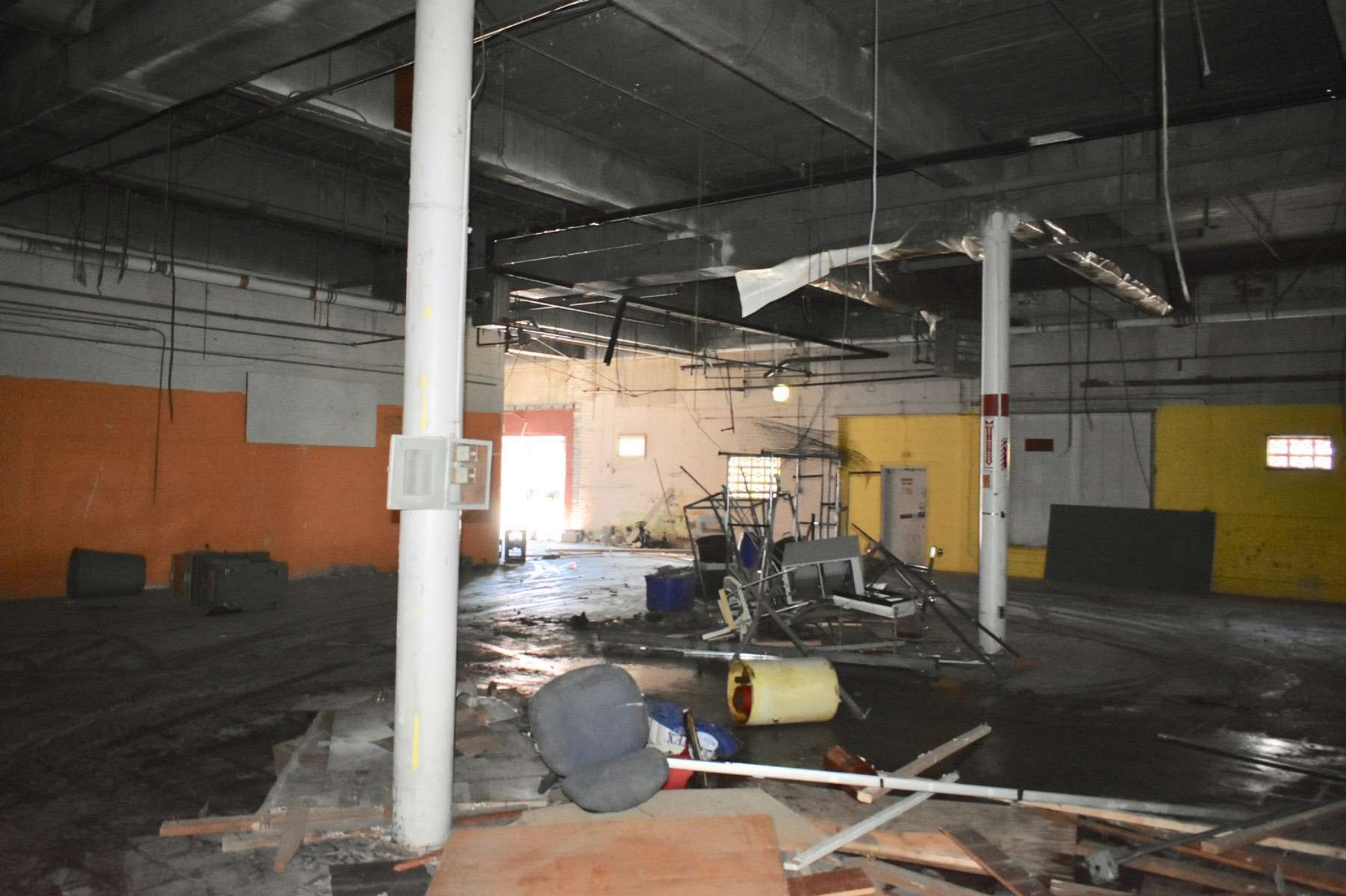
Photo #33 Building 3: Phillips Baker Rubber Company Building, first floor facing southeast.
