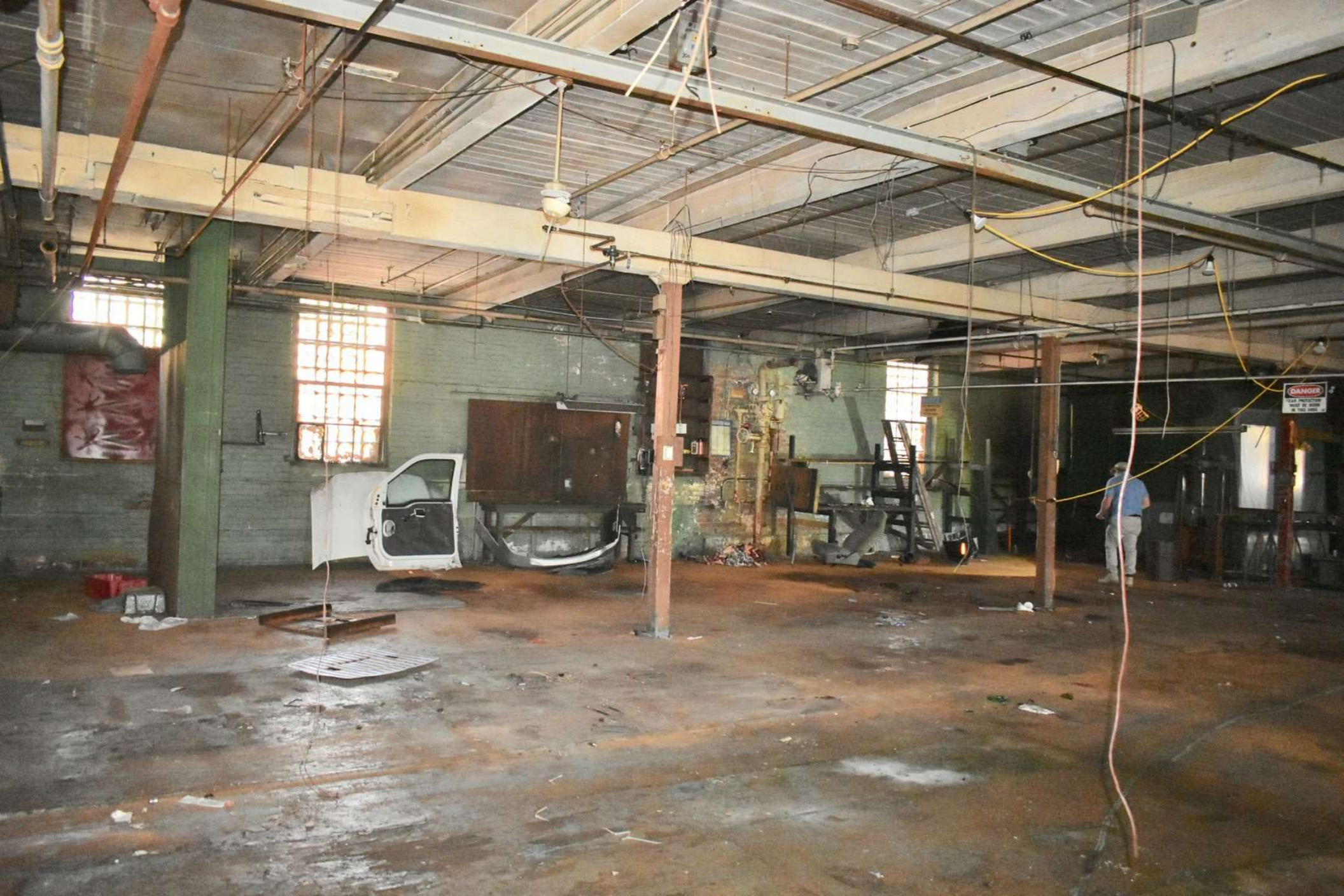
Photo #18 Building 2: Bourn Rubber Company Receiving Building, first floor facing northwest.
