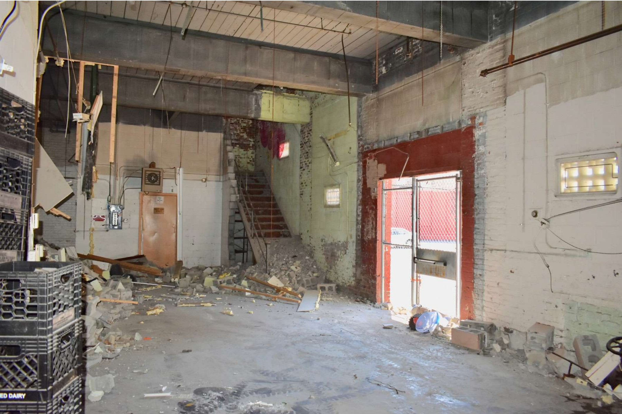
Photo #34 Building 3: Phillips Baker Rubber Company Building, first floor facing southeast.
