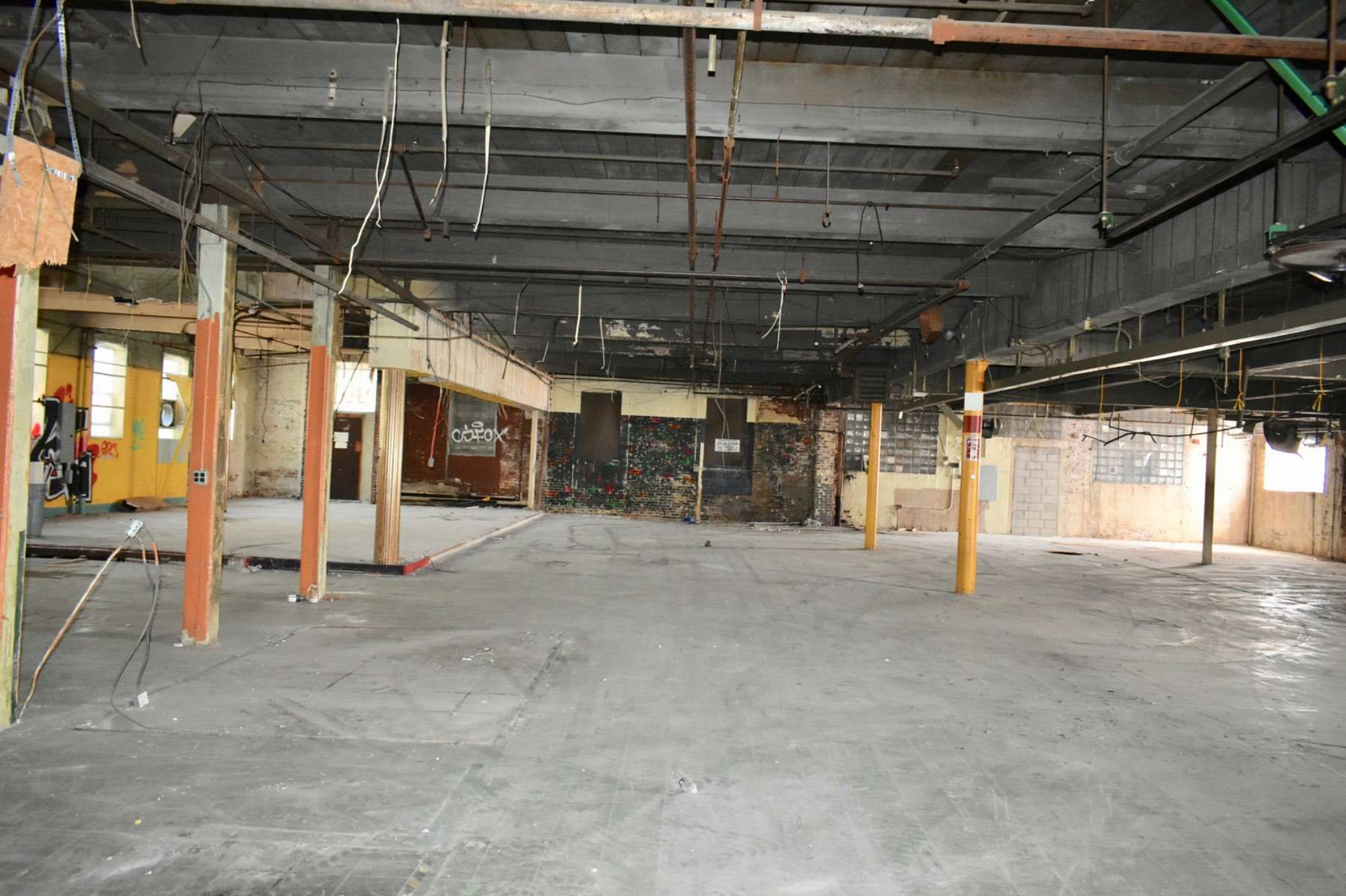
Photo #7 Building 1: Stedman & Fuller Manufacturing Company Building, first floor facing north.
