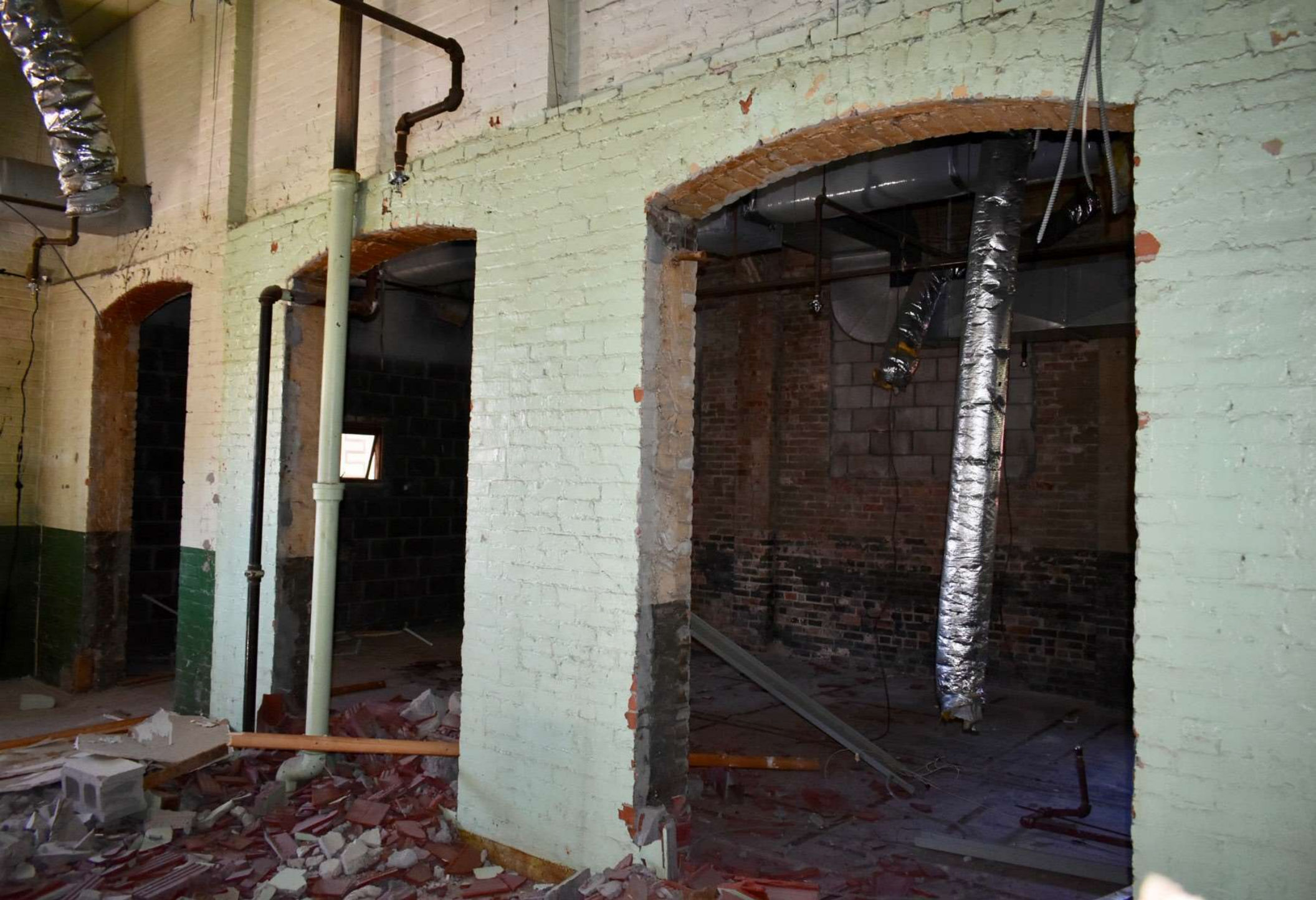
Photo #12 Building 1: Stedman & Fuller Manufacturing Company Building, second floor facing northwest.
