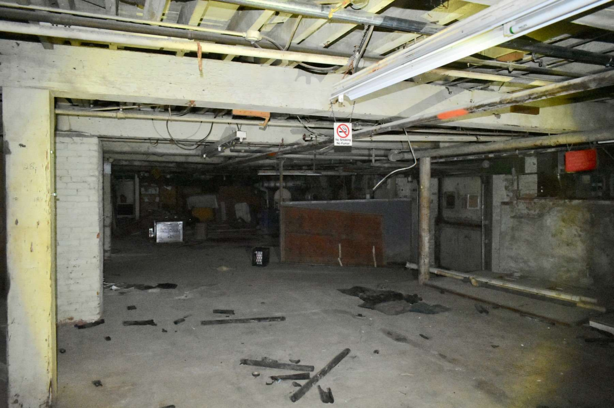
Photo #5 Building 1: Stedman & Fuller Manufacturing Company Building, basement facing southwest.
