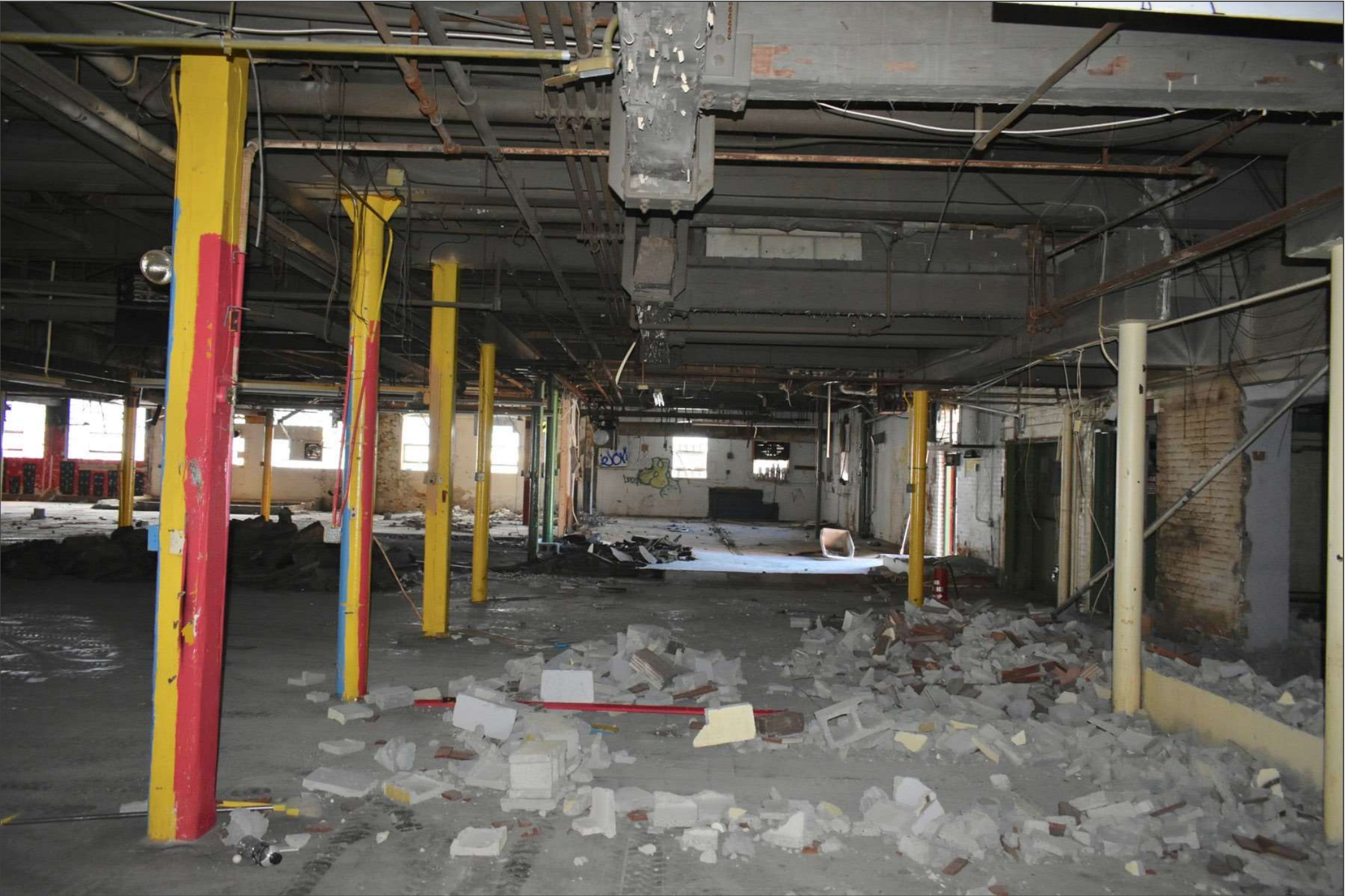
Photo #9 Building 1: Stedman & Fuller Manufacturing Company Building, first floor facing south.
