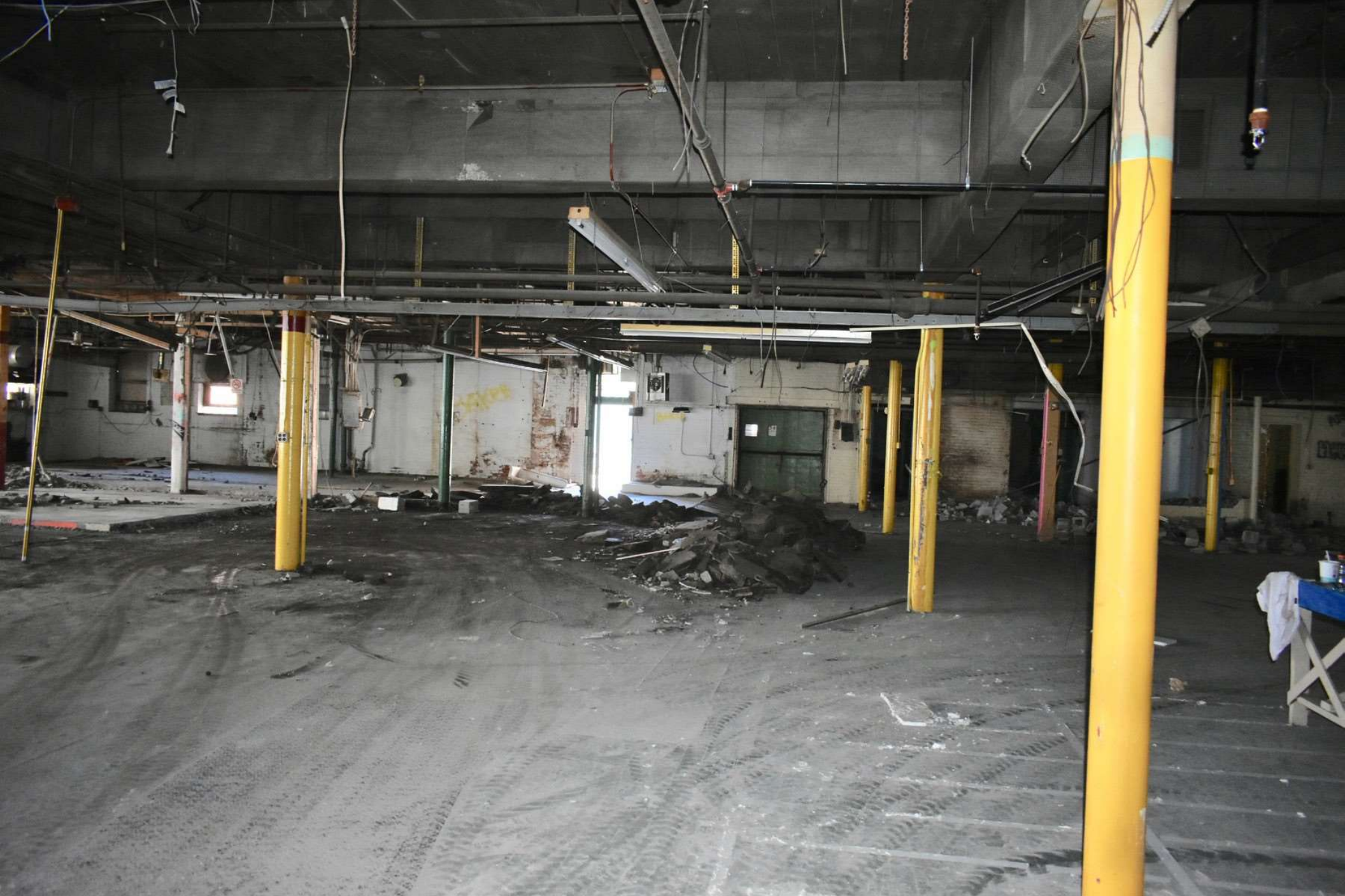
Photo #28 Building 3: Phillips Baker Rubber Company Building, first floor facing west.
