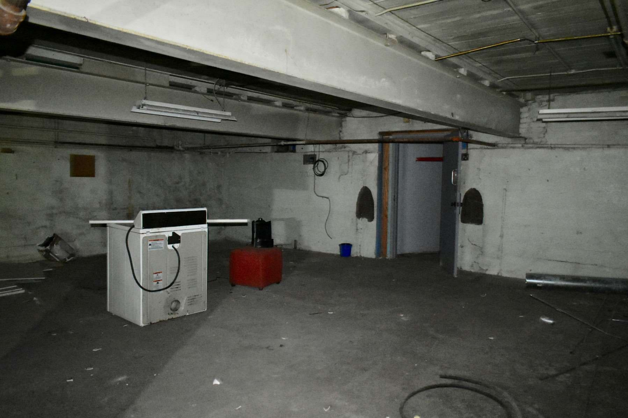
Photo #26 Building 3: Phillips Baker Rubber Company Building, basement facing southwest.
