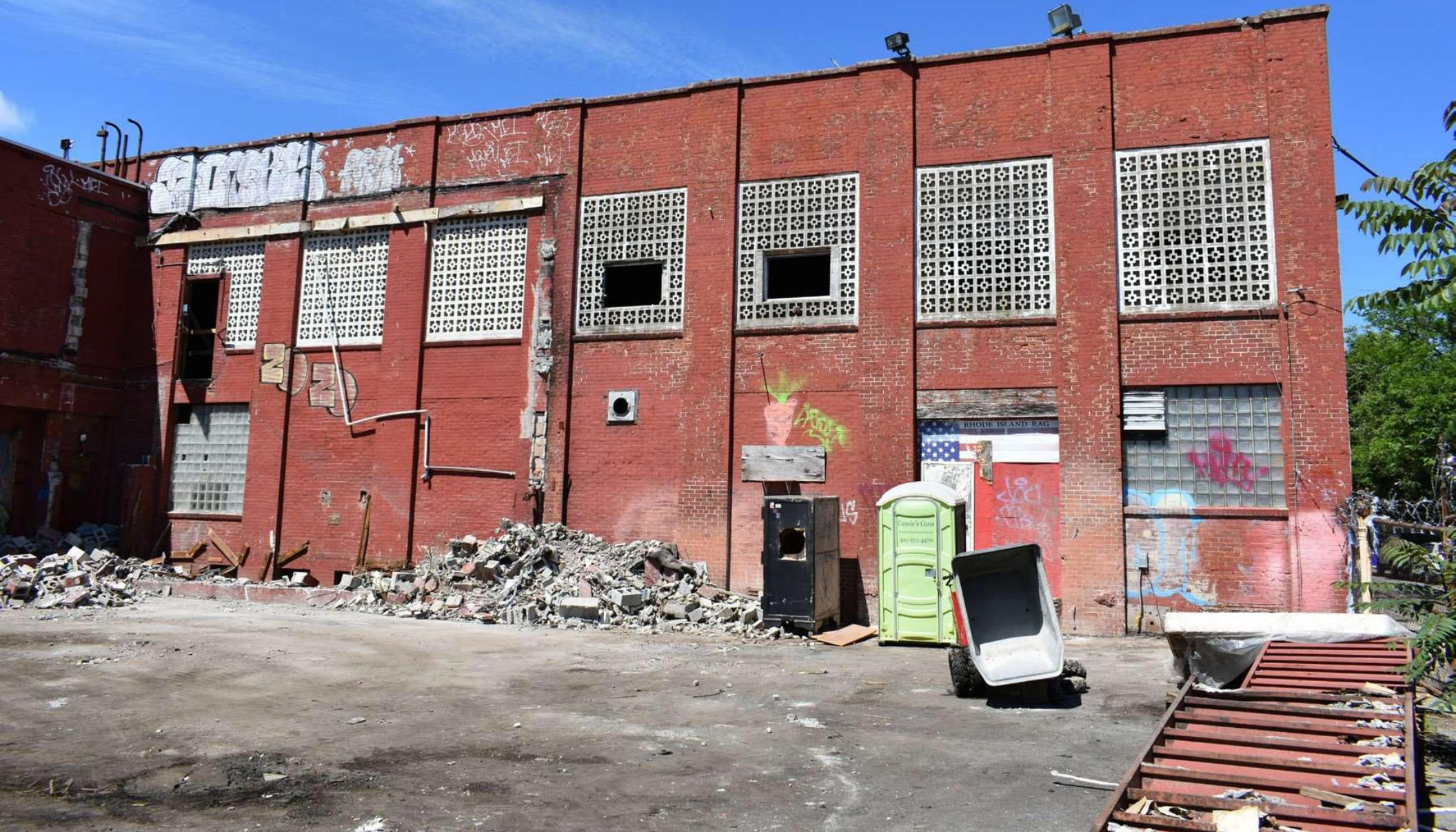
Photo #25 Building 3: Phillips Baker Rubber Company Building, east elevation facing southwest.
