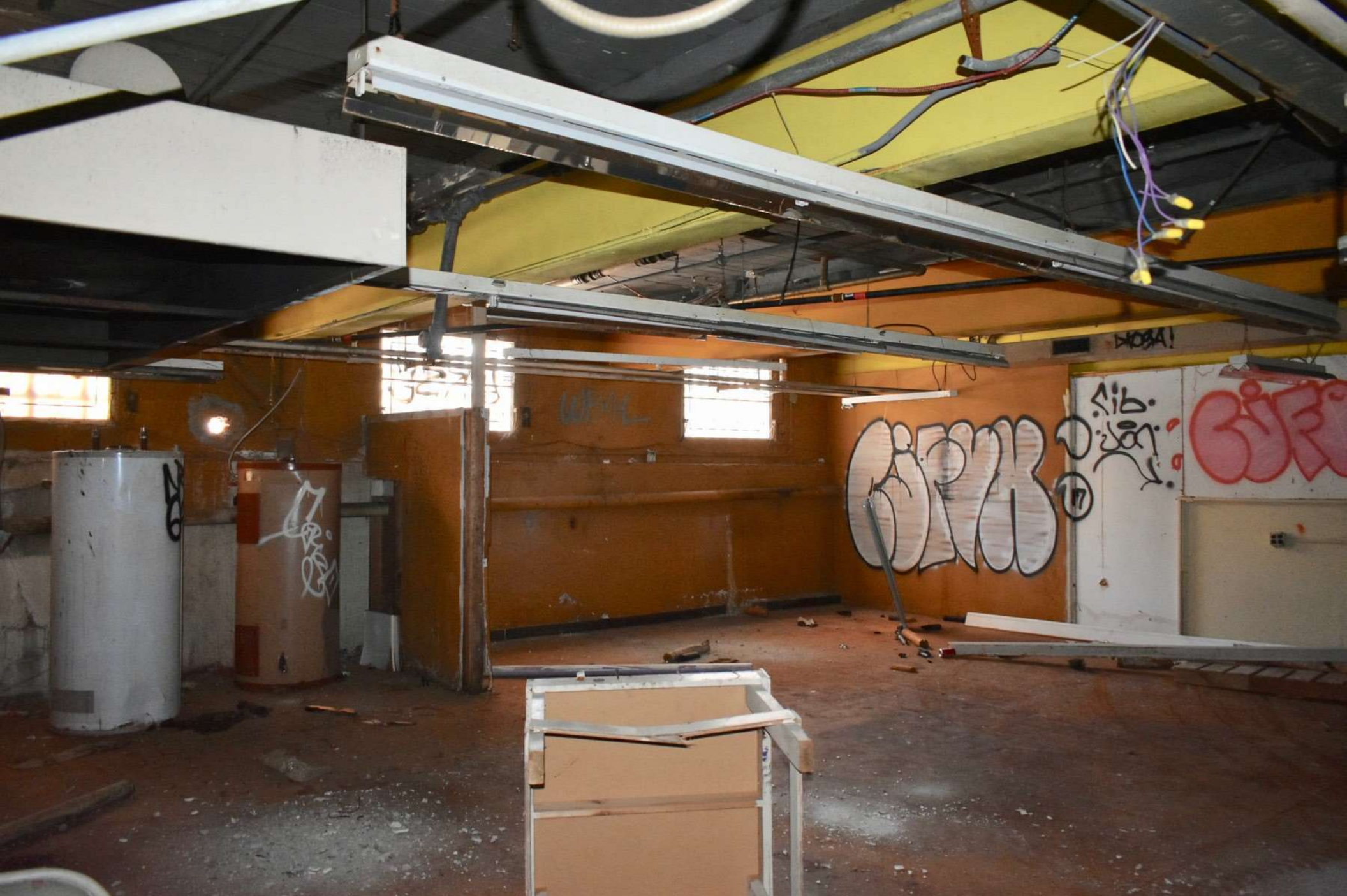
Photo #27 Building 3: Phillips Baker Rubber Company Building, basement facing southwest.
