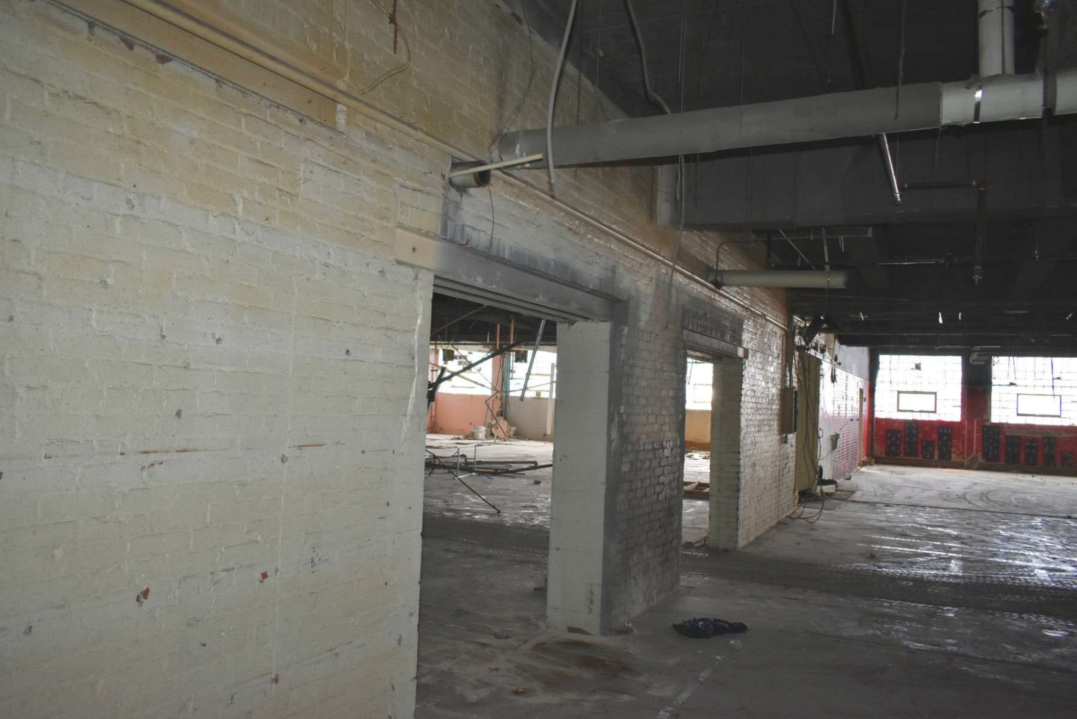
Photo #30 Building 3: Phillips Baker Rubber Company Building, first floor facing southeast.
