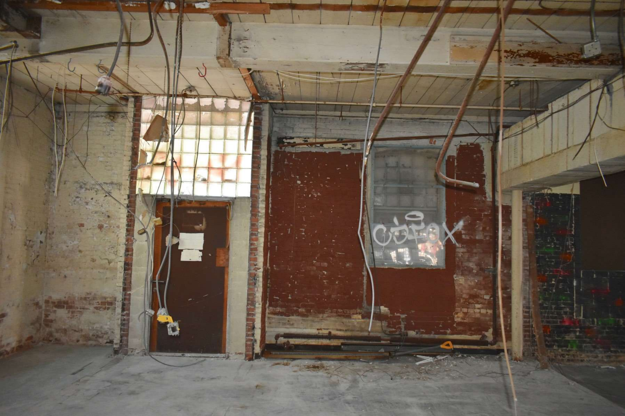
Photo #8 Building 1: Stedman & Fuller Manufacturing Company Building, first floor facing north.
