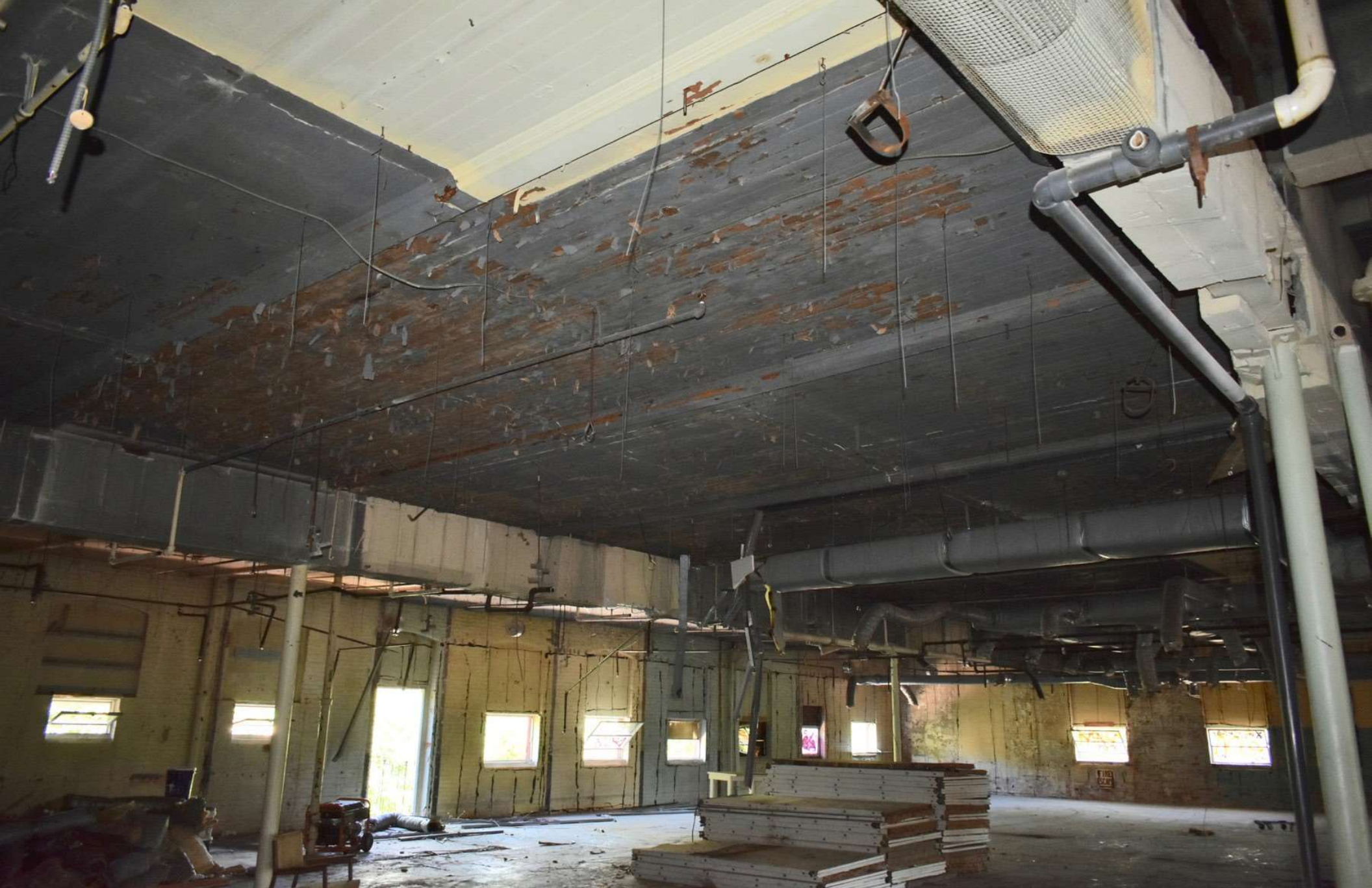
Photo #10 Building 1: Stedman & Fuller Manufacturing Company Building, second floor facing northwest.
