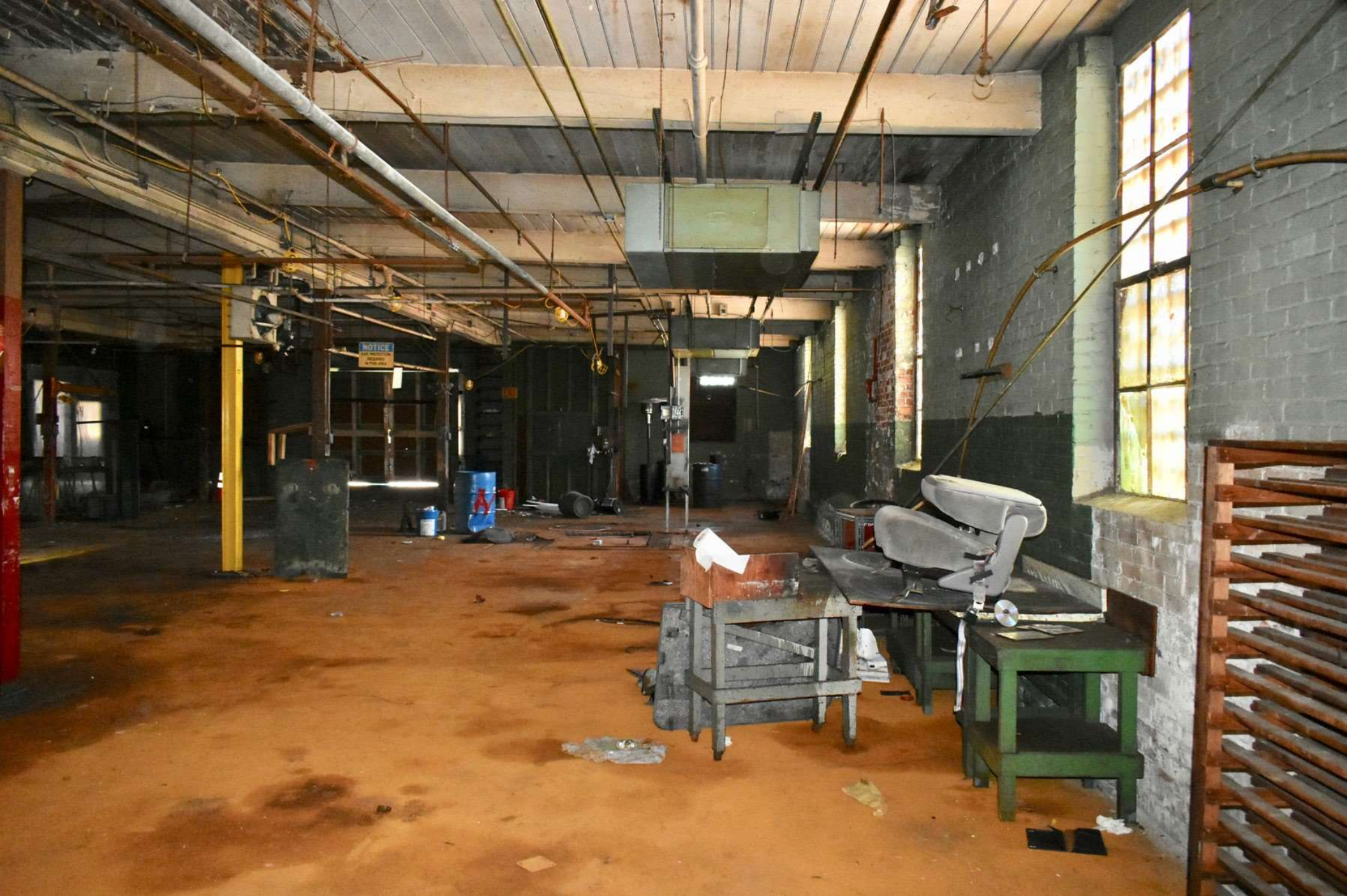
Photo #16 Building 2: Bourn Rubber Company Receiving Building, first floor facing north.
