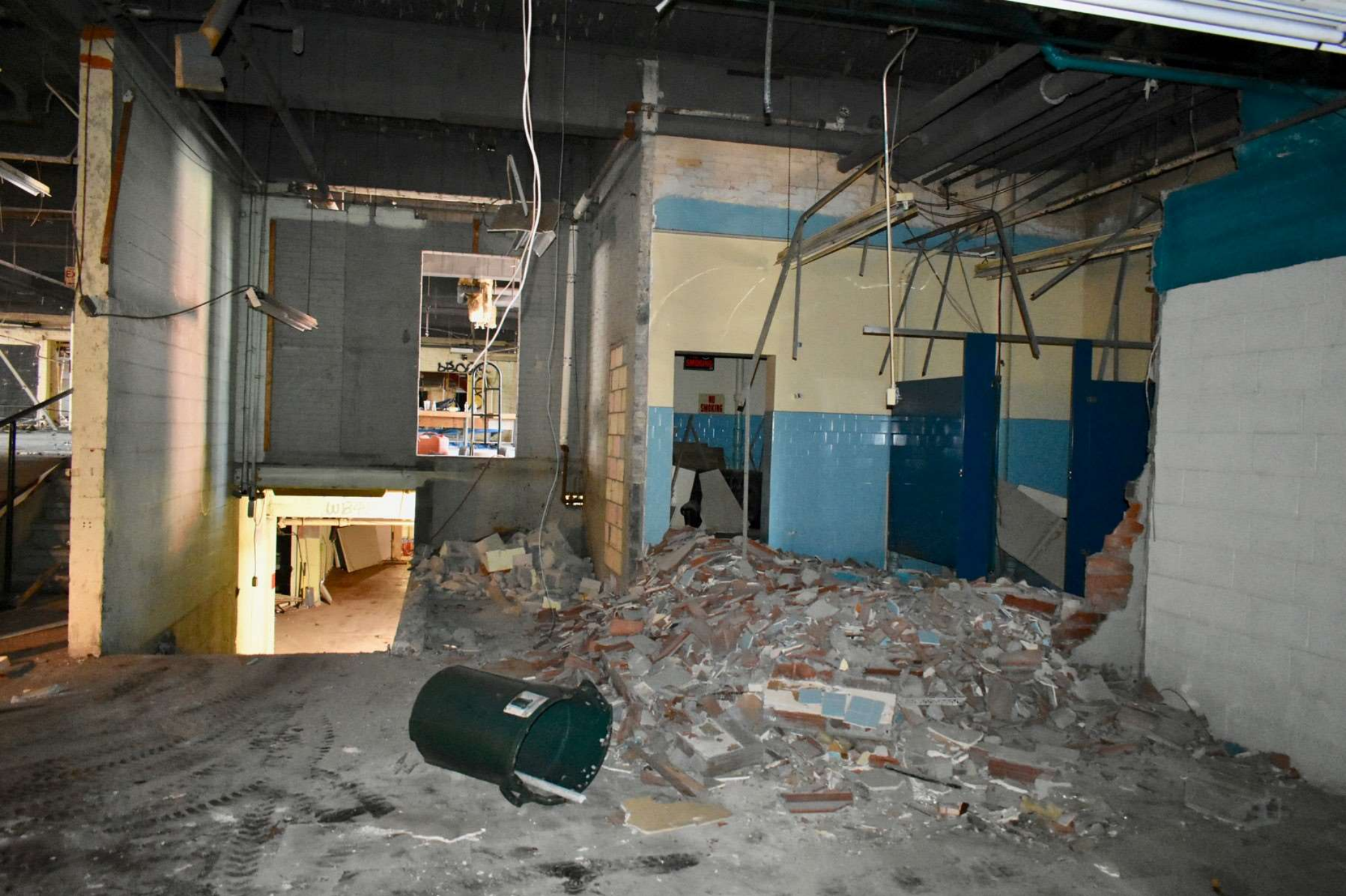
Photo #32 Building 3: Phillips Baker Rubber Company Building, first floor facing west.
