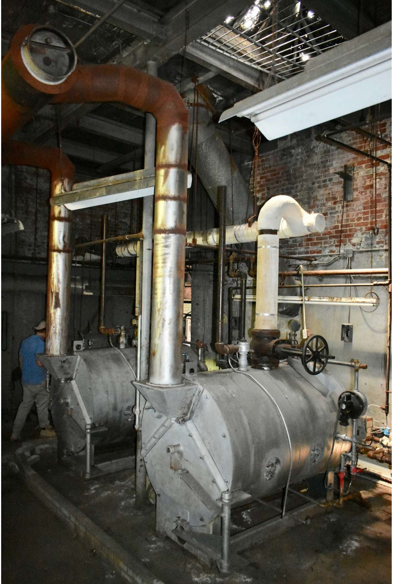
Photo #36 Building 3: Phillips Baker Rubber Company Building, first floor facing southeast.
