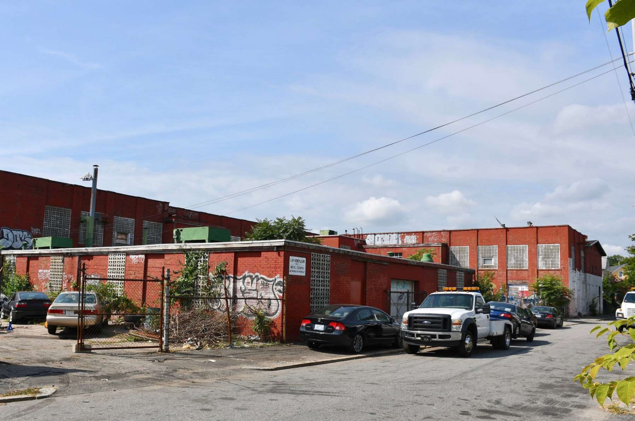
Photo #14 Building 2: Bourn Rubber Company Receiving Building (foreground), north and east elevations, facing southwest.
