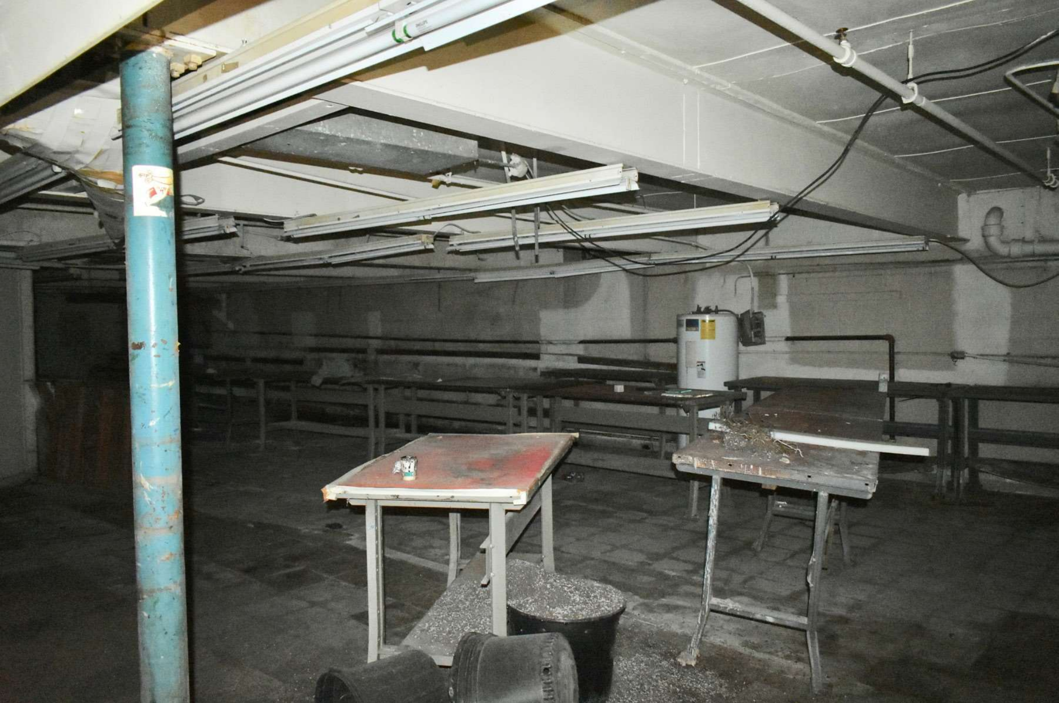
Photo #6 Building 1: Stedman & Fuller Manufacturing Company Building, basement facing southwest.
