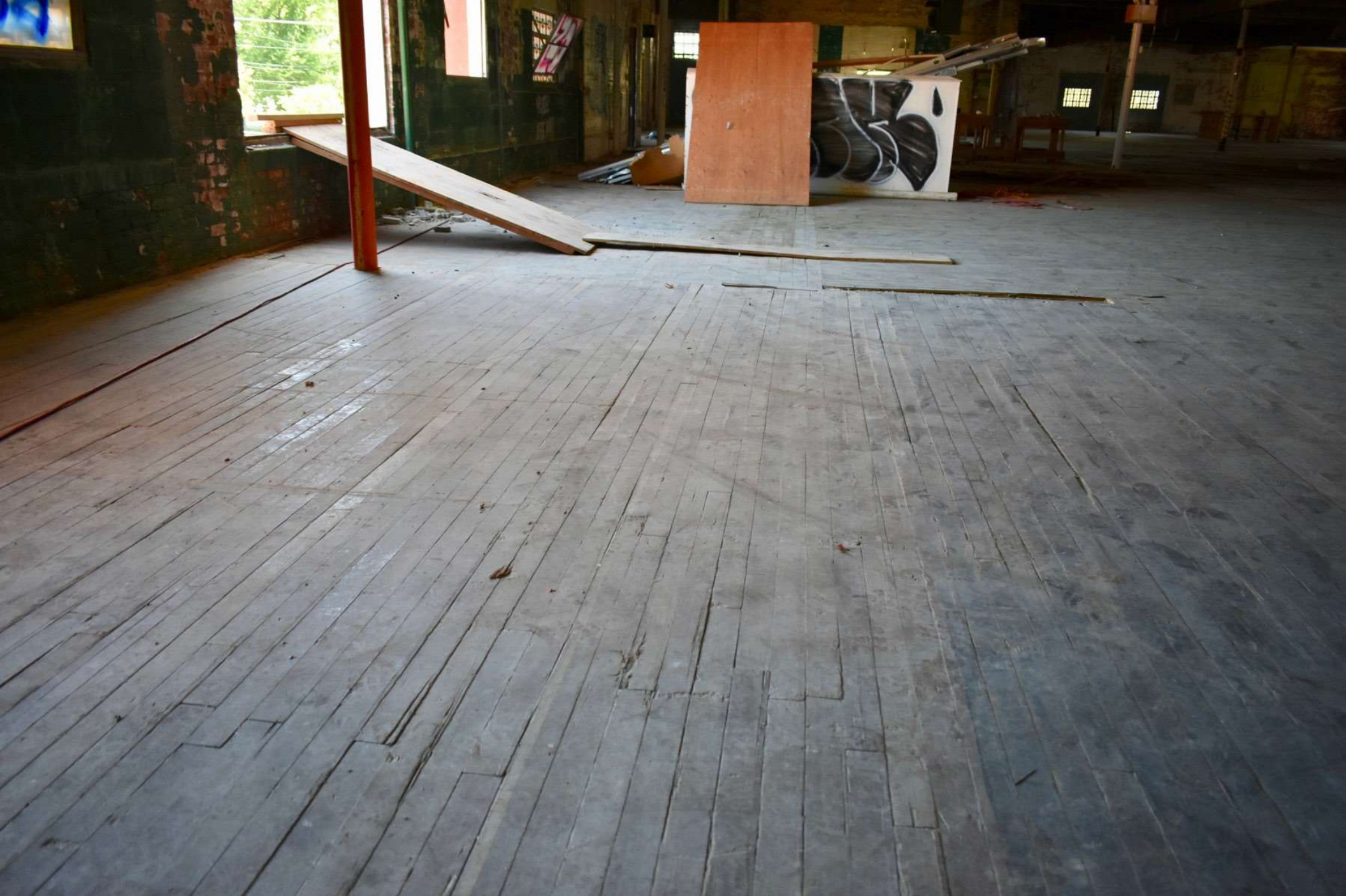
Photo #40 Building 3: Phillips Baker Rubber Company Building, second floor facing east.
