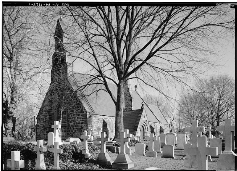
St. James the Less Episcopal Church, Philadelphia, Pa. (1846-48), based on drawings of St. Michaels, Longstanton by G.G. Place, supervising architect John E. Carver.
