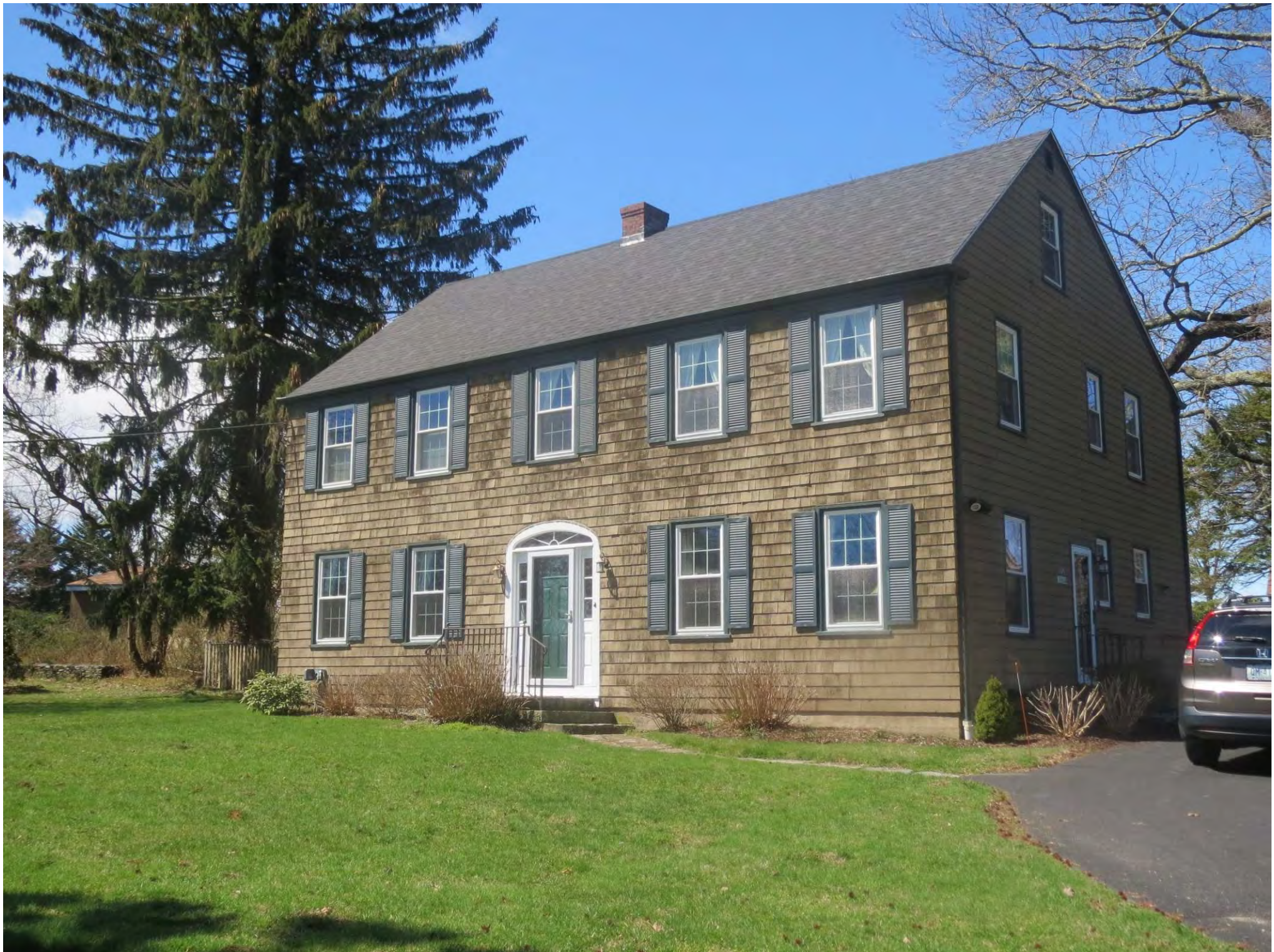
Photo #16: St. Mary's Rectory, east façade and north elevation, looking southwest.
