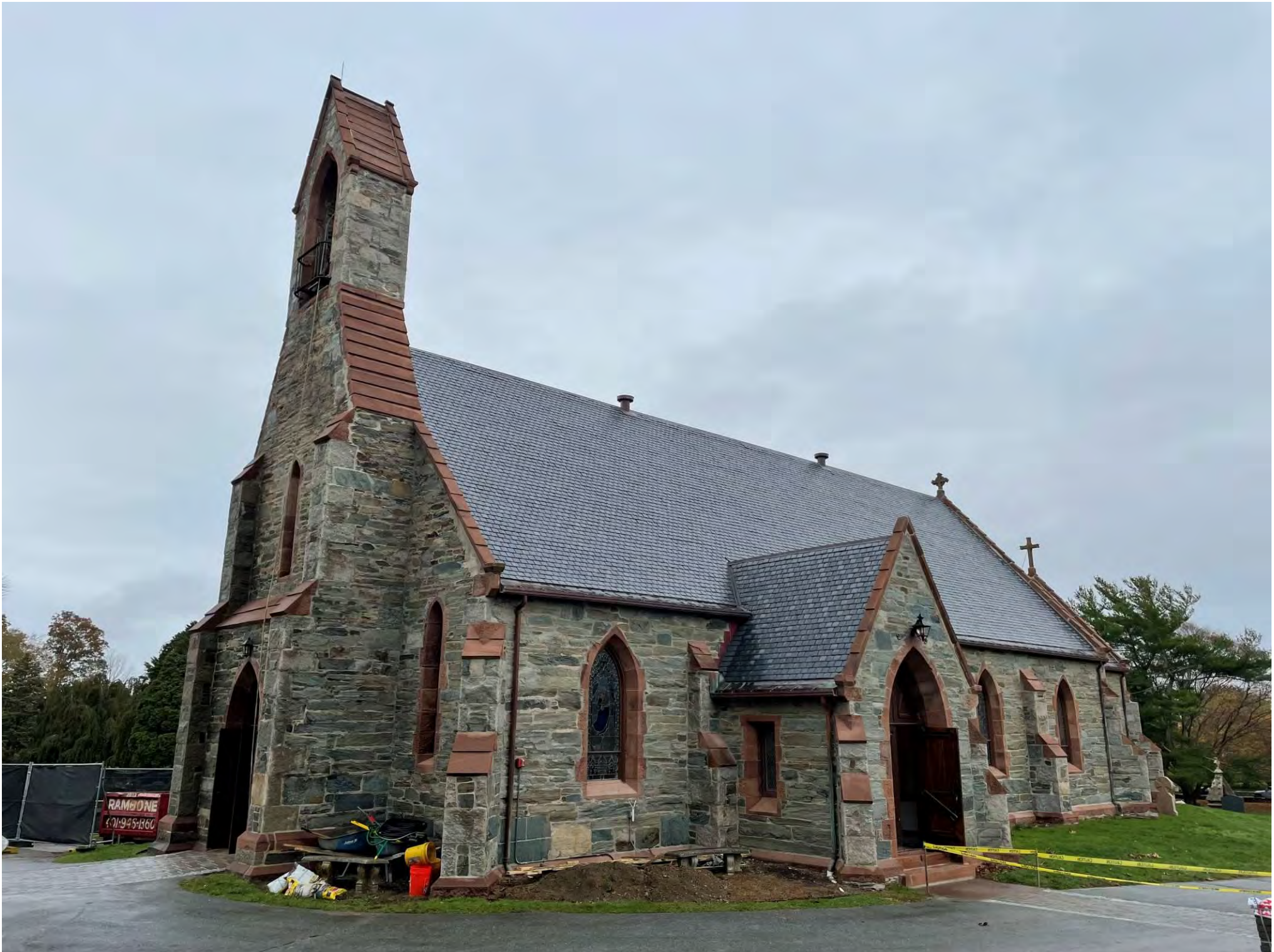
Photo #1: St. Mary's Church, west façade and south elevation, looking northeast.
