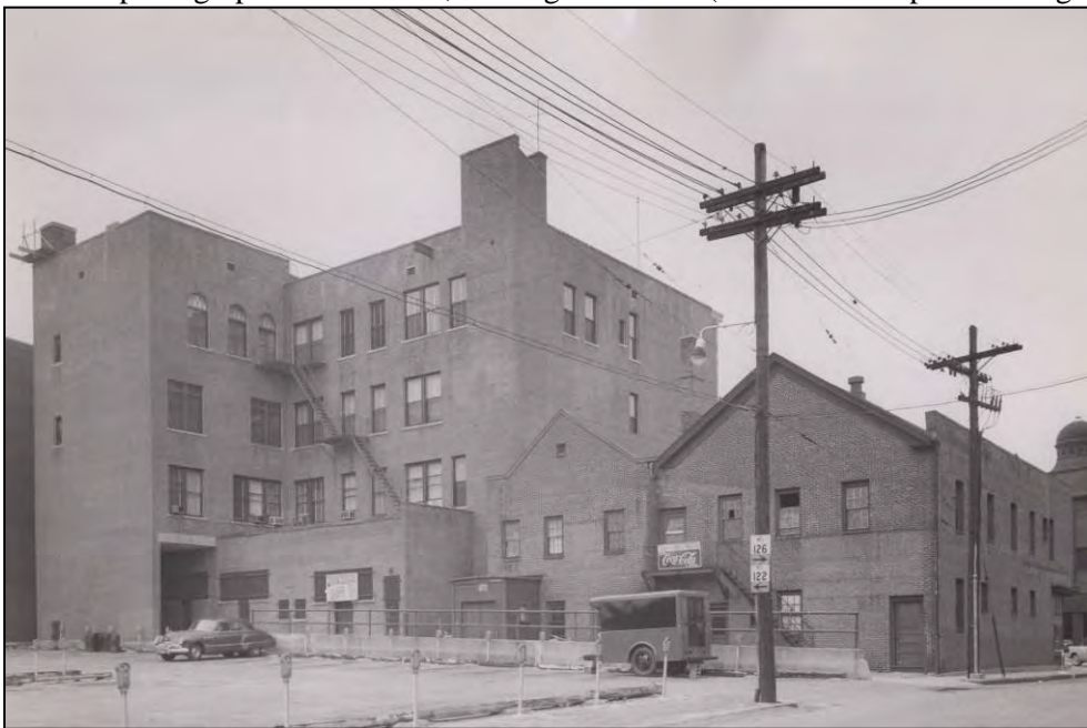
Undated photograph of rear of building prior to demolition of buildings on right and widening of street, looking northwest (source: Assumption College).
