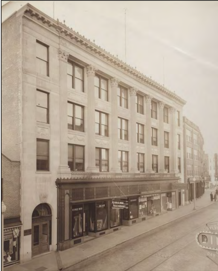
Undated photograph of the facade, looking southwest (source: Assumption College).
