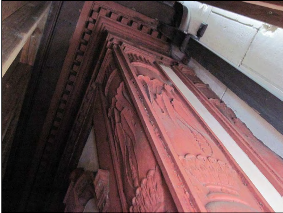
Detail photograph of the stamped sheet metal storefront beneath the pea stone soffit on the facade (Source: Aharonian & Associates Inc. 2017).
